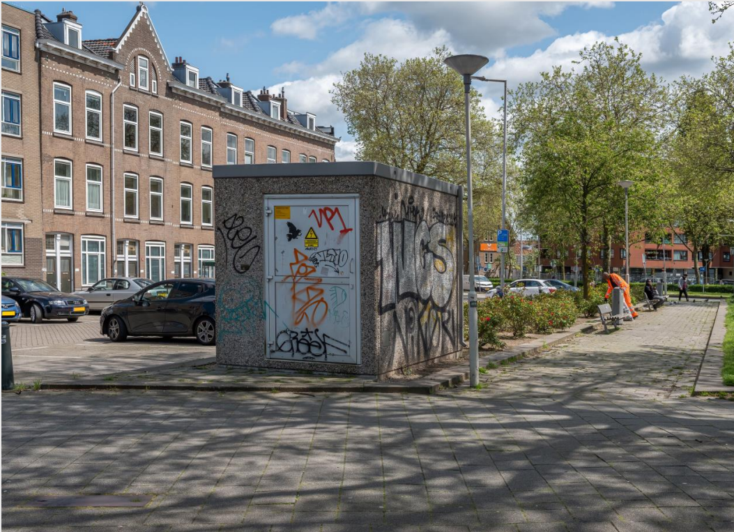
Forse betonnen behuizing
